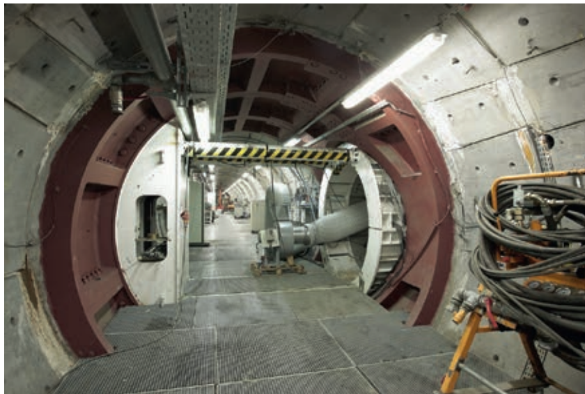
Figure 6 Support structure (white) at the entrance of the PRACLAY gallery
