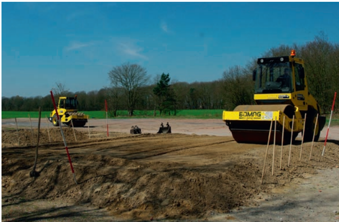
Figure 55 - V2 vibrating roller for tamping the sand (top left), and V2 sheep's foot roller (top right) for compacting the clay. In the bottom image, the vibrating roller was driven forwards and backwards over the sand tumulus during installation of a second sand layer.
