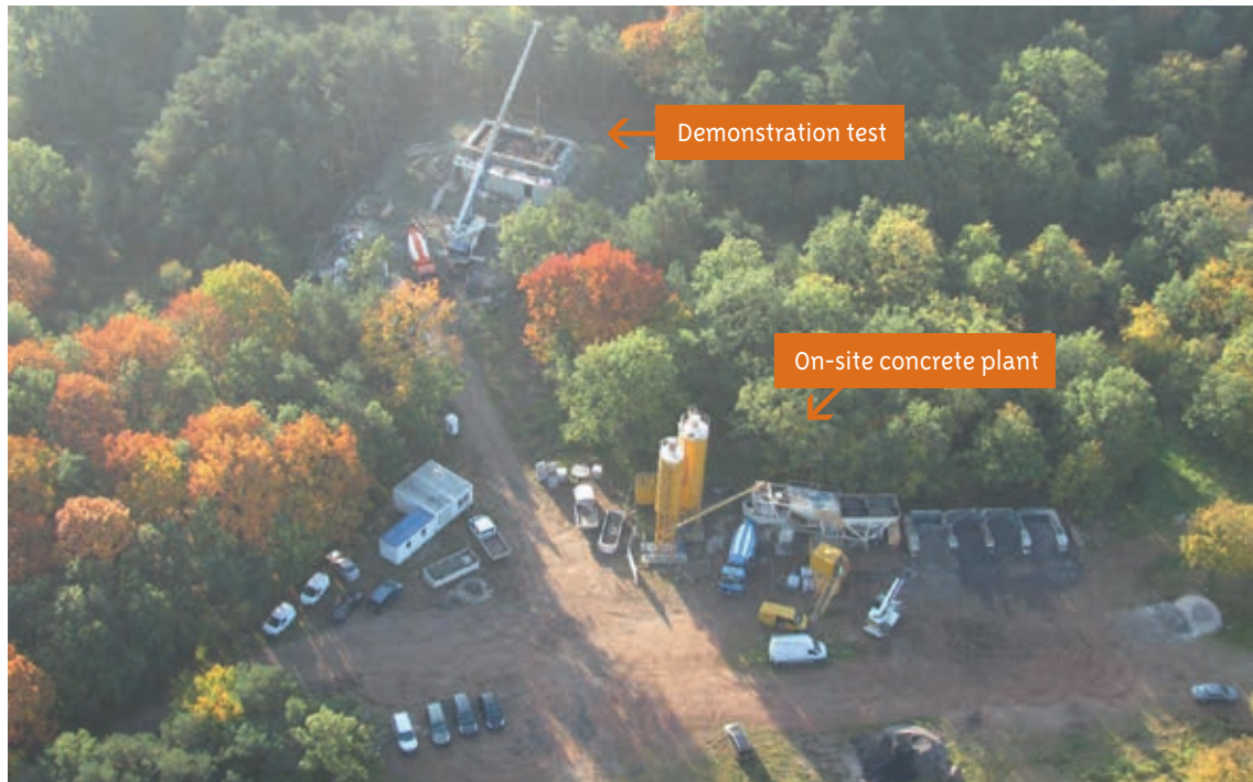
Figure 59 - Overview of the demonstration test
