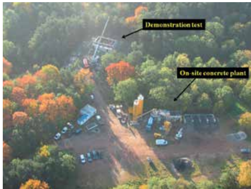
Figure 26 - Overview of the demonstration test
