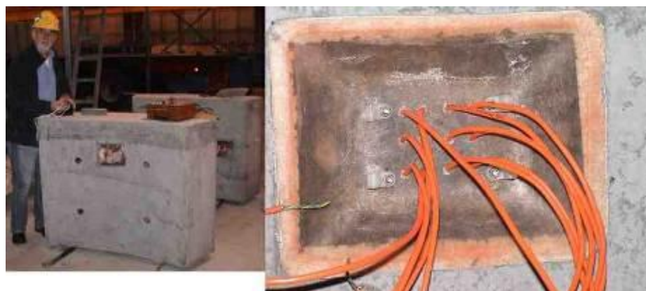
Figure 5.16 : View on the first two segments after unmoulding; detail (right) of the feedthrough shell after the protective sheet has been removed
