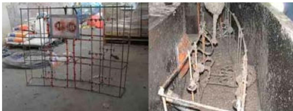
Figure 5.15 : Cage (12 gauge segment) just before and during concrete casting
