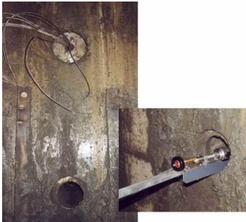
Figure 5.11: Original position of inclinometer E1, one meter under piezometer E2; optical and borehole camera survey (right).
