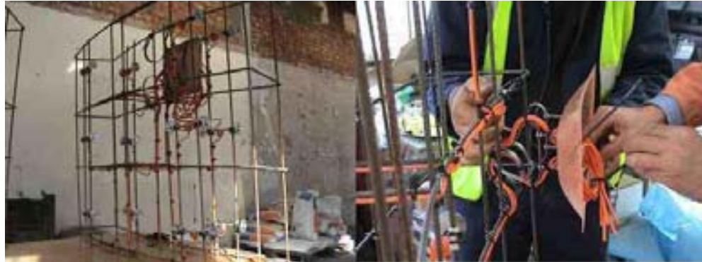
Figure 5.14 : Instrumented cage (left); detail of feedthrough shell (right)
