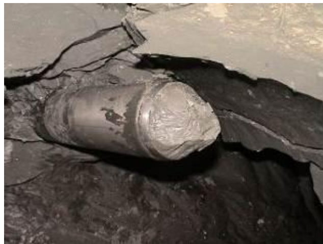
Figure 8.3: piezometer A2 uncovered at the excavation front
