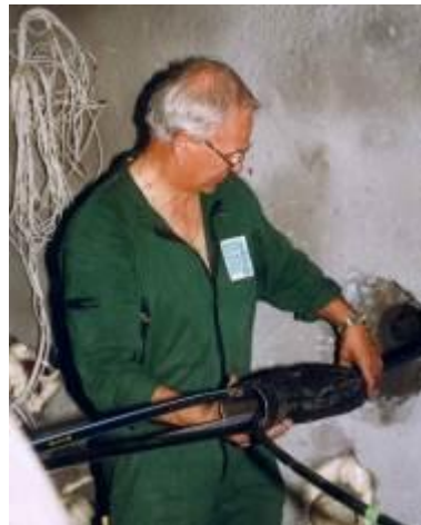
Figure 5.6: Installation of an extensometer anchor packer
