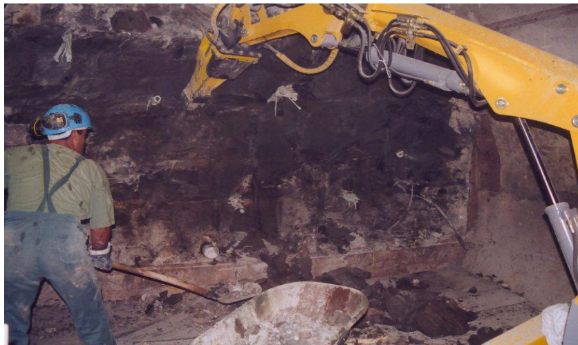
Figure 7.3: The start of the excavation of the mounting chamber
