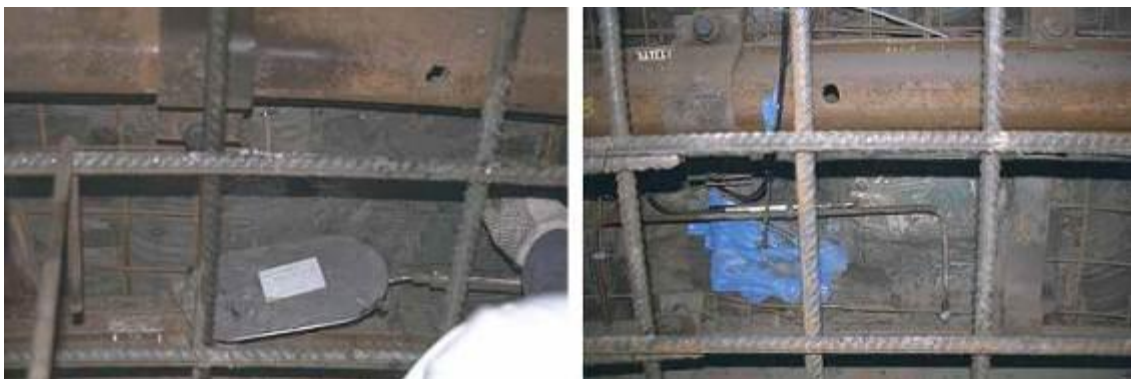
Figure 5.13: Preparation of the clay interface (left) ; installed sensor (sensor B3), before casting concrete (right)
