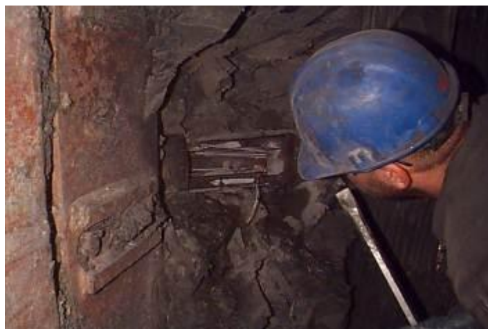
Figure 8.8 : Cutting of the D2 piezometer at the excavation front
