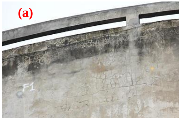
ASR at containment building of Tihange NPP (a) [FANC 2013], Seabrook NPP (b) [Saouma et al. 2014] and cemented waste drum from Doel NPP (c) [FANC 2014]
