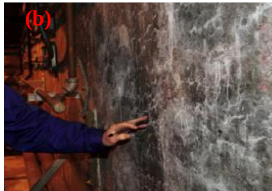
ASR at containment building of Tihange NPP (a) [FANC 2013], Seabrook NPP (b) [Saouma et al. 2014] and cemented waste drum from Doel NPP (c) [FANC 2014]
