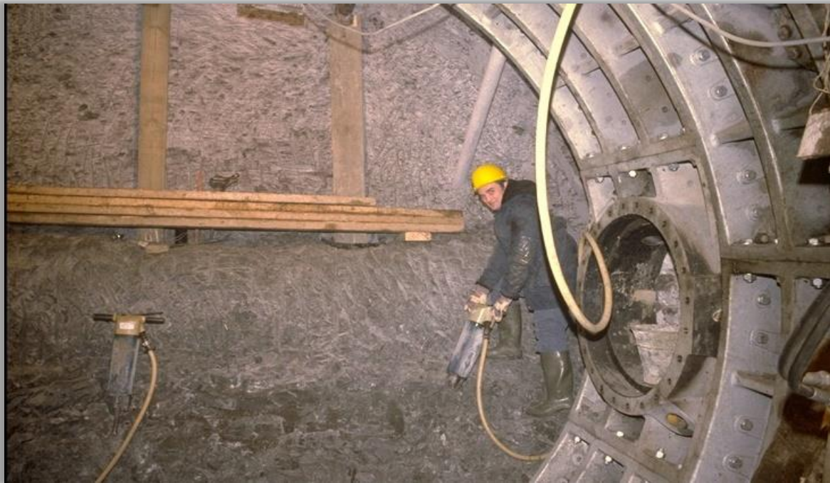
Semi-manual excavation in frozen clay
