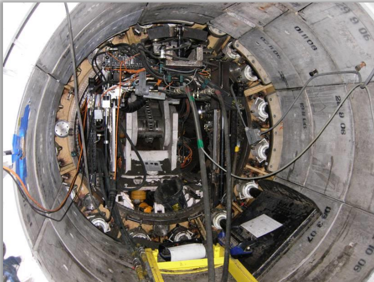
3. Gallery lining emplacement
