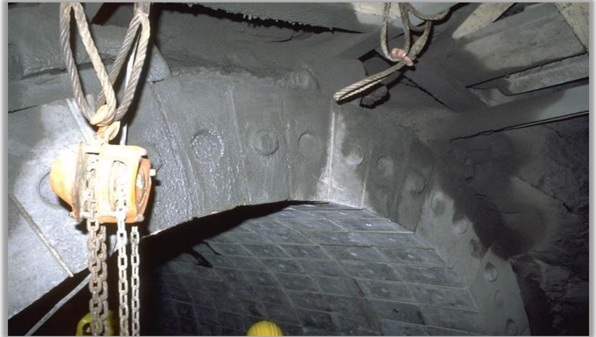
Lining: concrete blocks & wood plates
