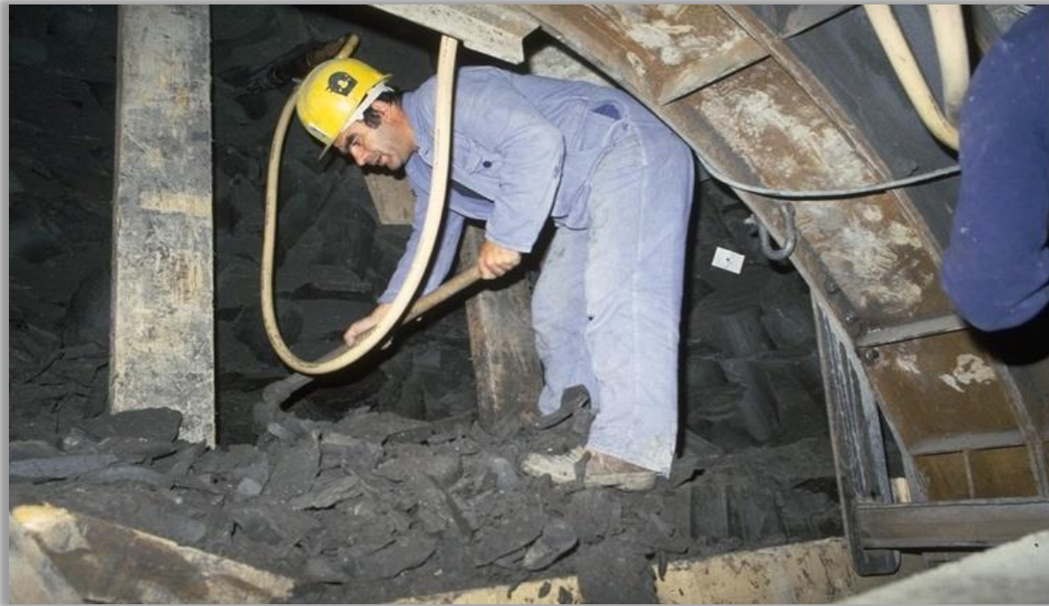
Front: (semi-)manual excavation
