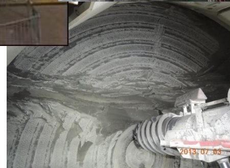
Road header under shield
