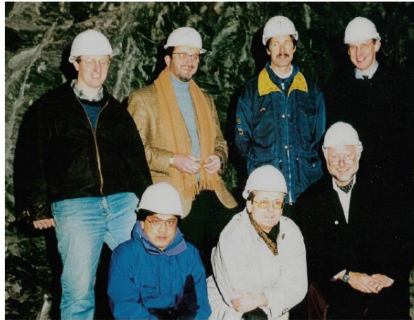
Start of niche excavation in 1996
