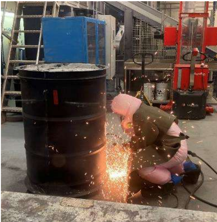
Removal of drum
