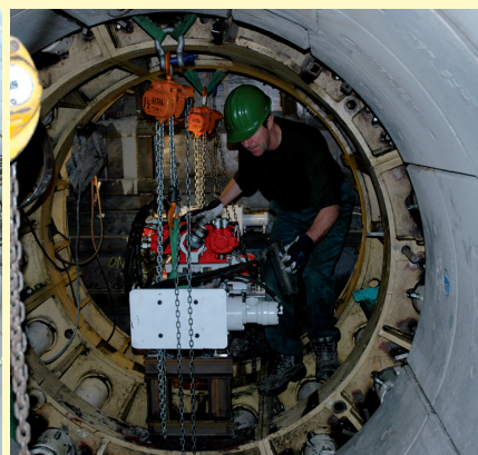
Boring in de Boomse klei
